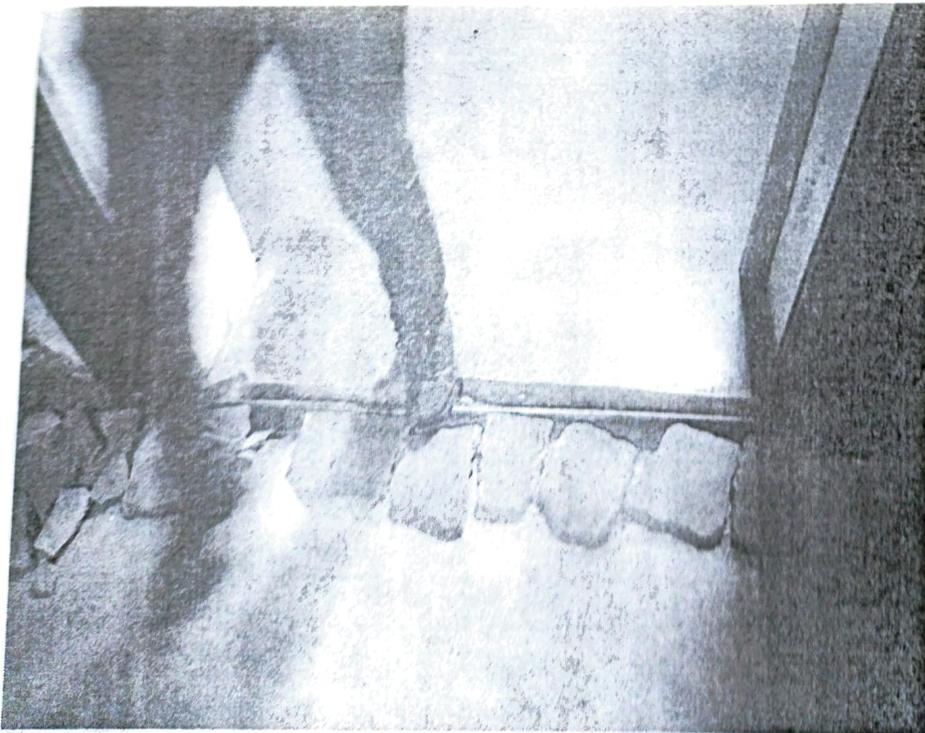
**Step ramp was Broken at the entry gate to hospital building from basement side (parking area)**
