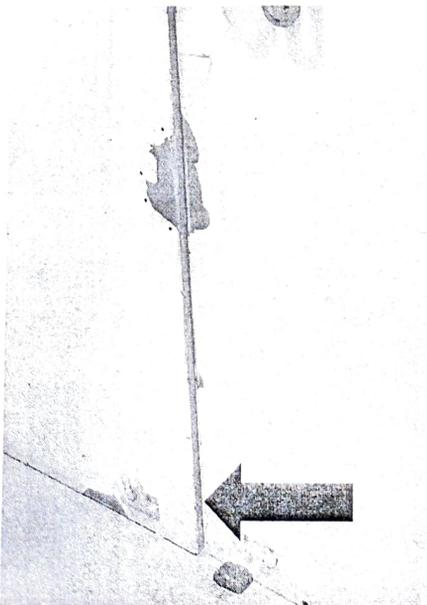
The door of SPECT room has gaps when closed completely and needs repair
